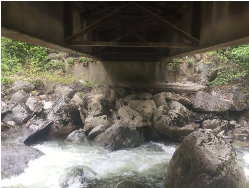
Left Bank Abutment when facing downstream
