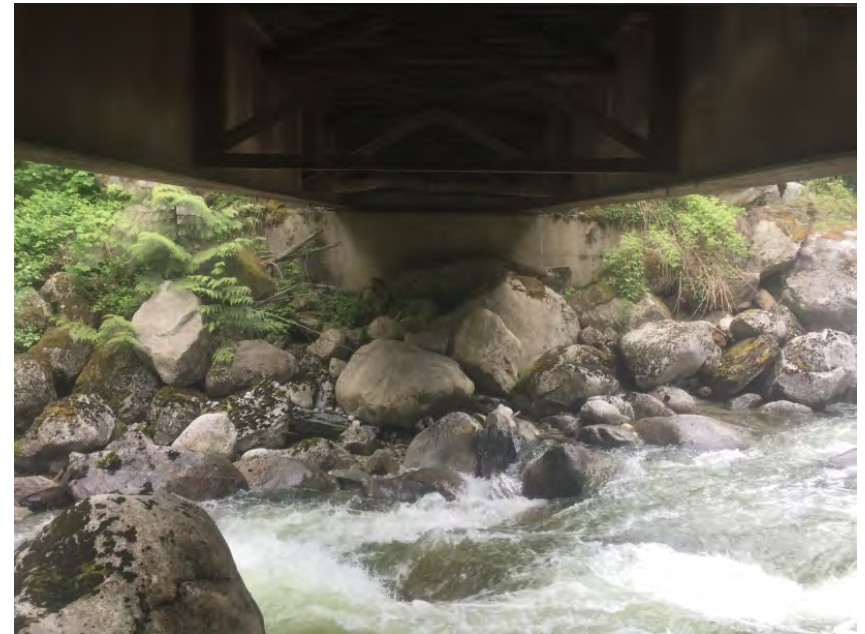
Right Bank Abutment when facing downstream
